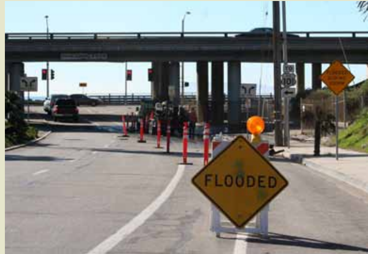
Fig. 6.29. San Jon Road at Highway 101, looking west. Areas of the Pierpont lowland are still susceptible to flooding, as shown in this December 2008 photograph.
