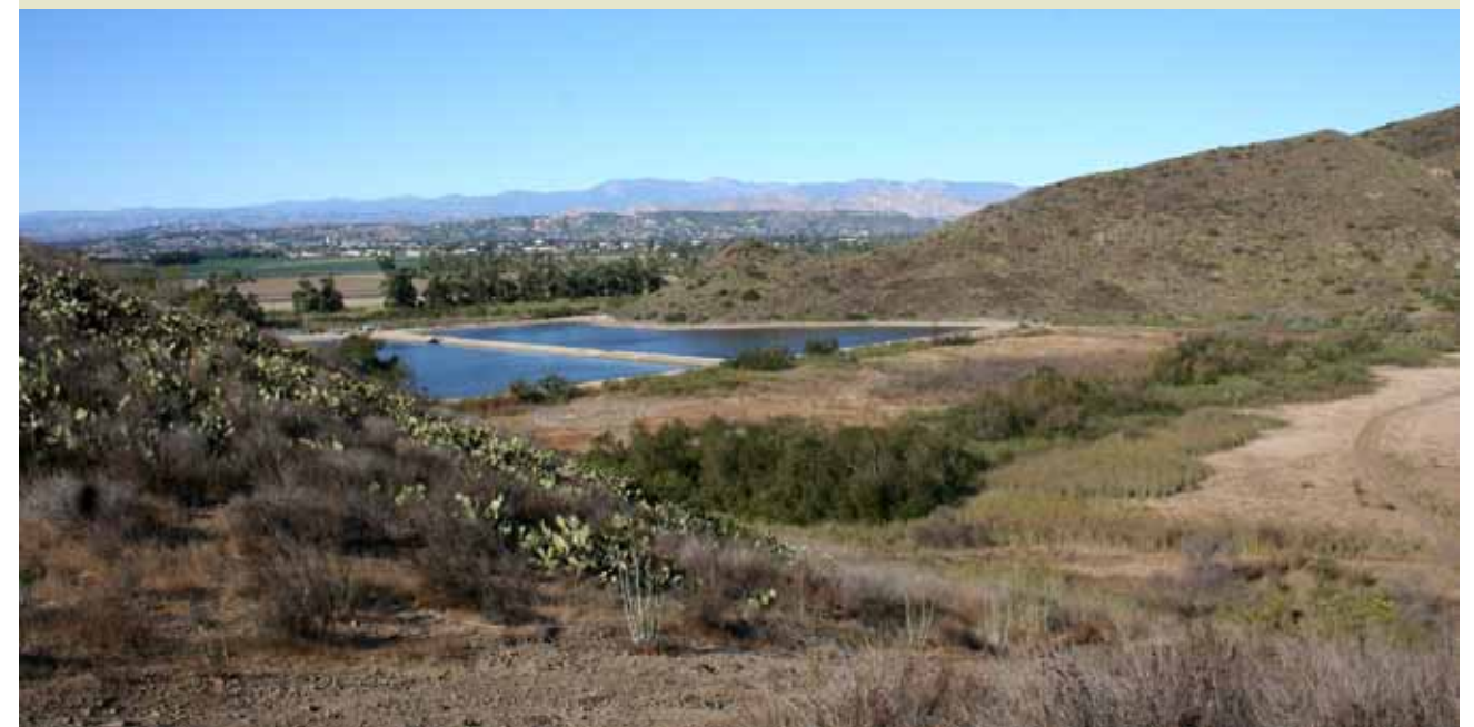
Fig. 5.17. Camrosa Water District storage ponds, 2008. The area behind these storage ponds, formerly the site of a freshwater marsh complex, may be a potential location for wetland habitat restoration.
